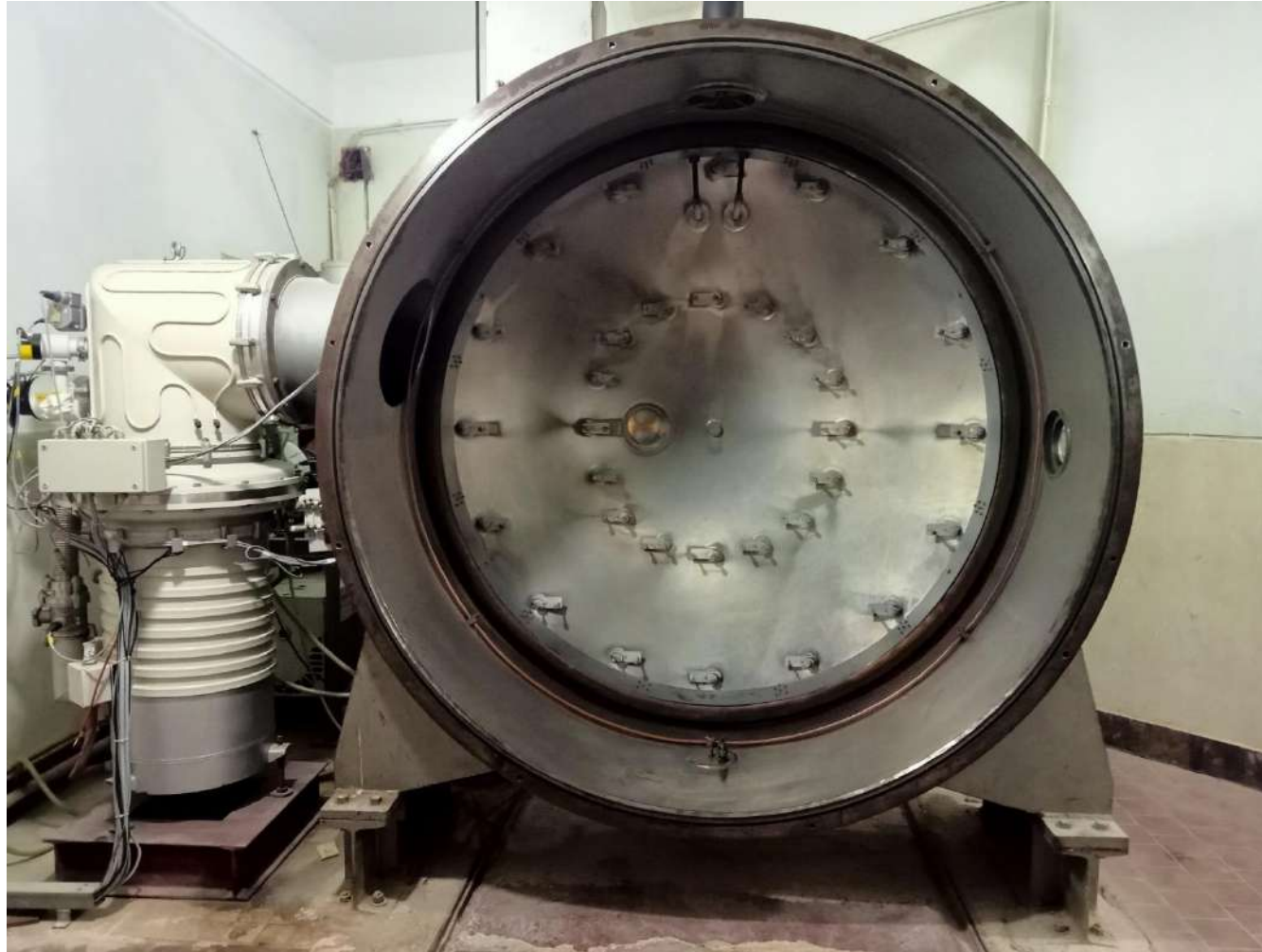
Internal view of the Aluminizing Plant
